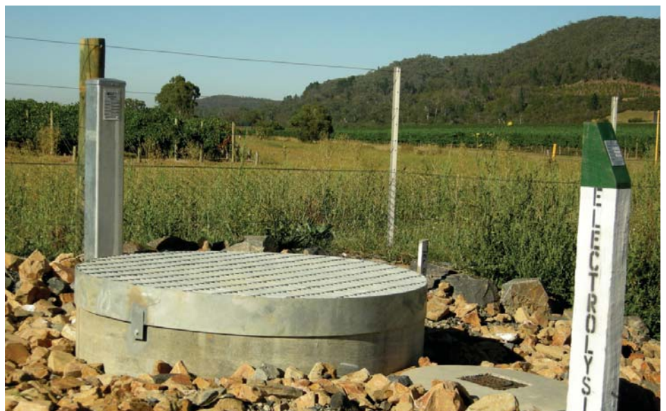
A scour valve (with marker bollard) and cathodic protection marker post near Yarra Glen
